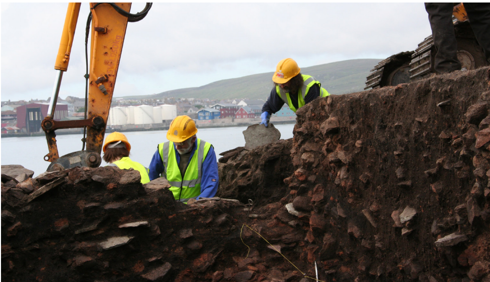
Figure 10: Local volunteers helping to move stone from the original site, Cruester
