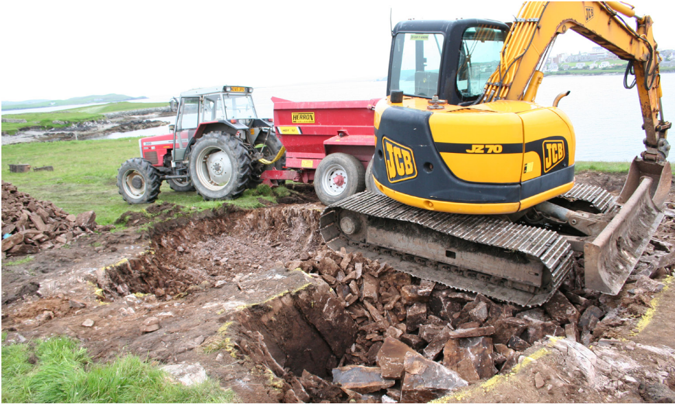
Figure 9: Precision digging within the painted lines at the reconstruction site, Cruester
