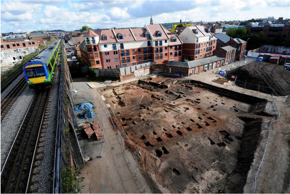
Figure 2: The Roman site looking towards the city of Worcester
