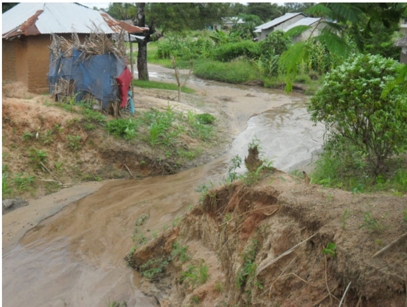
Figure 6: A water run-off through the demolished colonial railway. (Photo by the Author).
