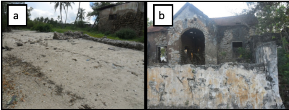
Figure 5: Erosive activities at Mvita site (a) and deteriorating monuments (b) at Mikindani historical site. (Photo by the Author).
