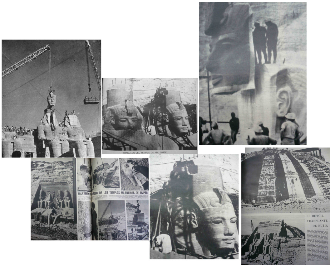
Fig. 8. Different moments and sequences of different stages of current work. Operators are fitting the face of Ramses II. 1963 © Arriba.
