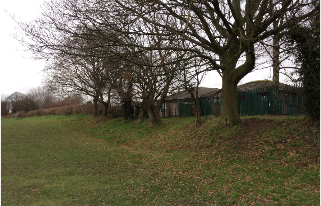
Figure 8: Wat’s Dyke in the Wrexham suburbs where it now constitutes the western boundary of Wat’s Dyke Primary School. Looking north in this photo, the bank is clearly preserved beneath the hedge and fence while the ditch is broad and shallow but discernible (Photograph: Howard Williams, 2019)
