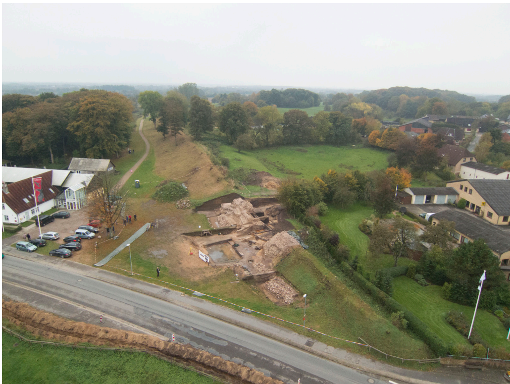
Figure 3: The excavation site in 2013 as seen from the east. The Main Rampart of the Danevirke runs from south-west to north-east. Today it is crossed by a modern road named 'Ochsenweg'. At the excavation site one can see the remains of the Fieldstone Wall, which has a wide gap, which is the site of the former gate. There is also the section through the Main Rampart (for details see Figure 6).
