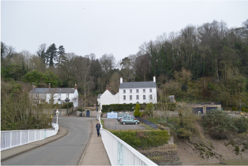
Figure 3: Chepstow Bridge (an early iron bridge across the Wye built by the engineer John Rastrick in 1816) looking north. The bank of Offa's Dyke occupies the top of the break of slope north from the bridge (above the houses on either side of the ancient routeway). Early in 2020, the co-authors traced the bank of the Dyke surviving in good condition ascending the slope diagonally from the roadside opposite Elm Villa up through the grounds of Castleford House to a point overlooking the cottages at left in this view (Photograph: Keith Ray)
