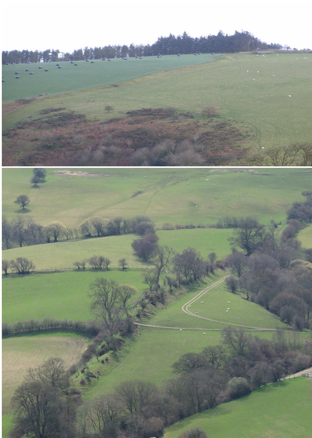
Figure 2: The Offa's Dyke 'adjusted-segmented' design/construction device. 2a (above): at Rushock Hill, Herefordshire. 2b (below): at Spoad, Newcastle-on-Clun, Shropshire (Photographs, left: Keith Ray; right: Adam Stanford)
