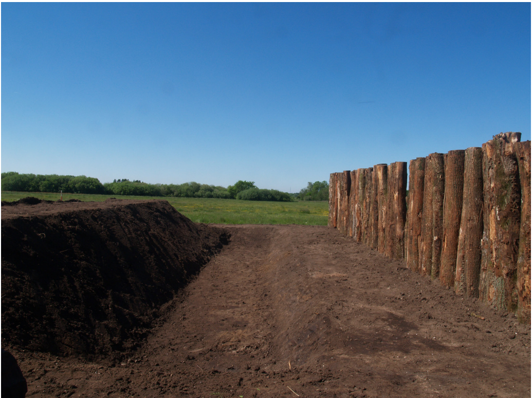
Figure 12 (below): Reconstruction of the Olger Dyke at Olmersvej 2021 (palisade, ditch and bank, viewed from the north). The photo was taken during the phase of reconstruction (Photograph: Lisbeth Christensen)
