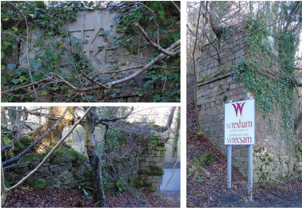
Figure 8: The nineteenth-century tower and wall marking Offa’s Dyke, Craignant, Shropshire/Wrexham (Photograph: Howard Williams, 2017)
